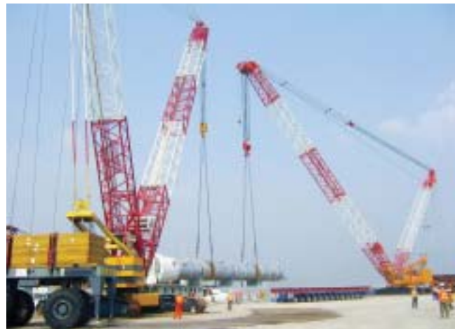
Our 550-ton and 300-ton heavy cranes performing a tandem lift at the Marine Offloading Facility in Nanhai, China.
